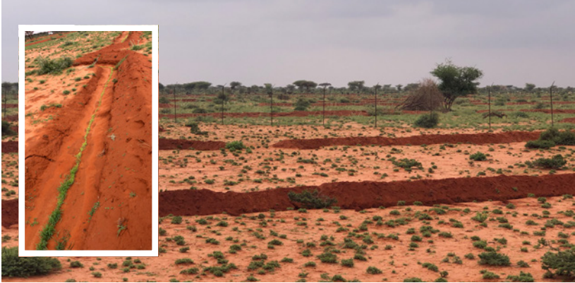
Newly constructed soil bunds, Nasiye, 2022. Source: The HALO Trust Somaliland
